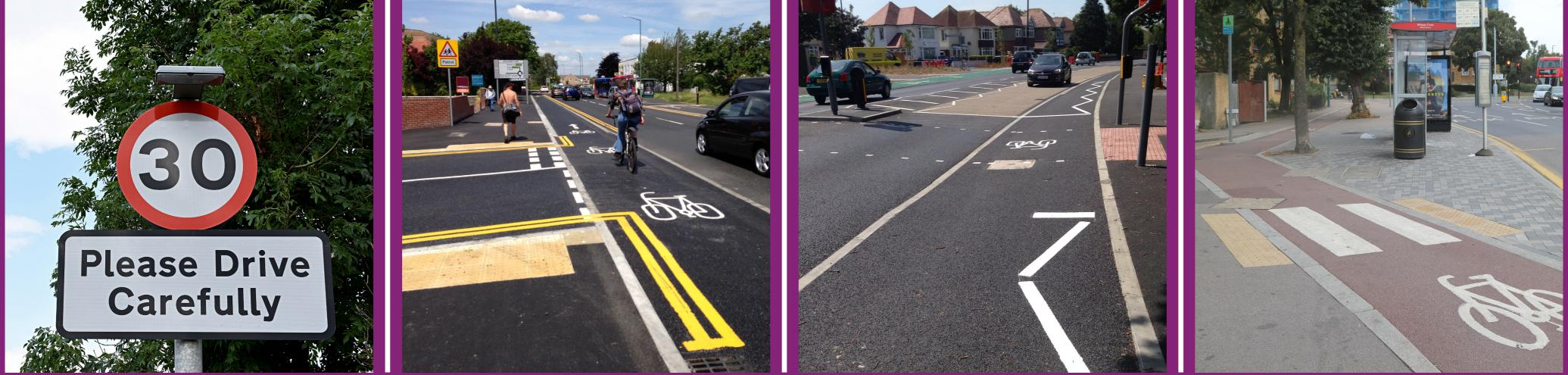
New bus stop layouts, with the cycle track routed behind them to separate motor traffic from cyclists. Informal zebra crossings would be installed to give bus users priority over cycle.
